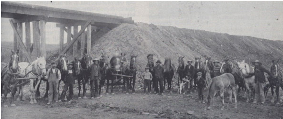
A construction gang near Minto
